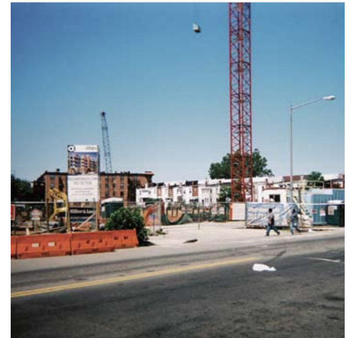
Figure 5: Park Place under construction
